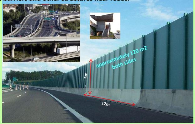
1 km of noise barriers with a height of 5m, which are painted on both sides FN, reduced for one day about 40% of the pollutants concentration of in the air volume of 700 to 900 thousands cubic meters. Price per coat − 131 000 €, functionality warranty - 10 years.
